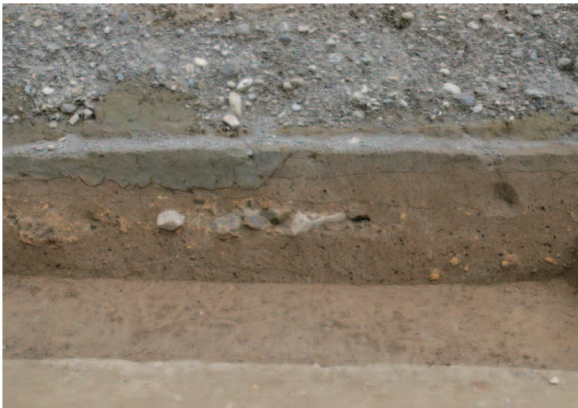
3-1区北壁土層堆積状況①
